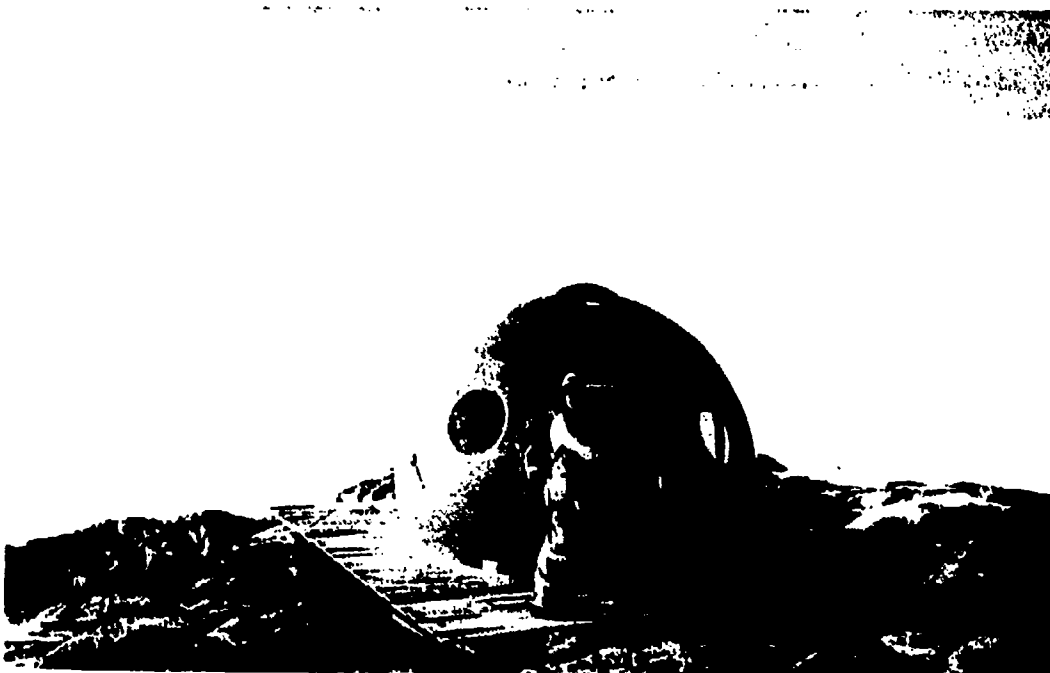
A light, transportable pre-fabricated fibreglass dome used by field parties (Antarctic Division, Australia).
